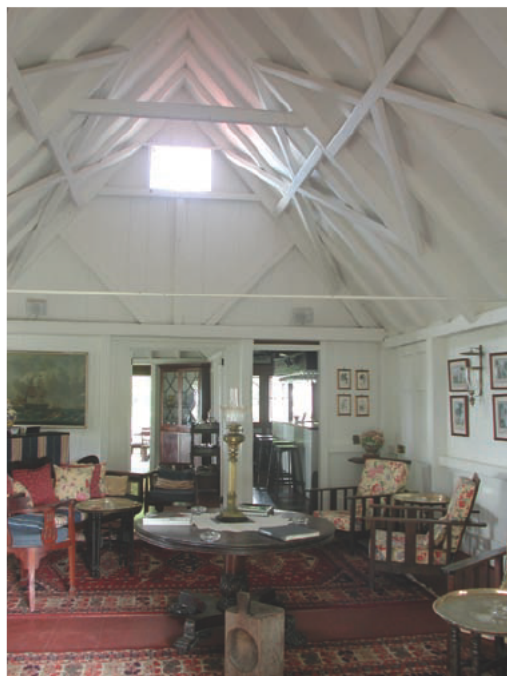
The open hall looking west (RHL)
