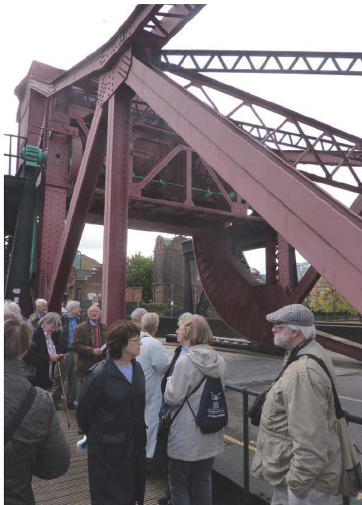
Shadwell Basin – the bridge gear (AB)
