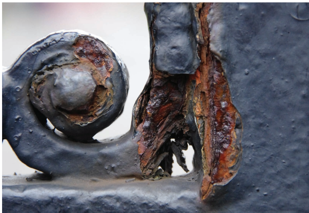
Failure of coating and subsequent corrosion of gates, Palace of Holyroodhouse, Edinburgh (NE)
